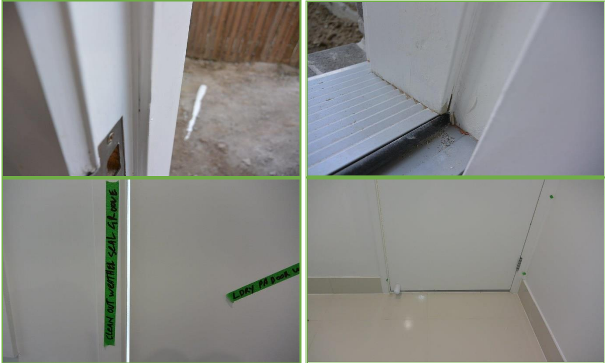
Allowing water to ingress during rain
