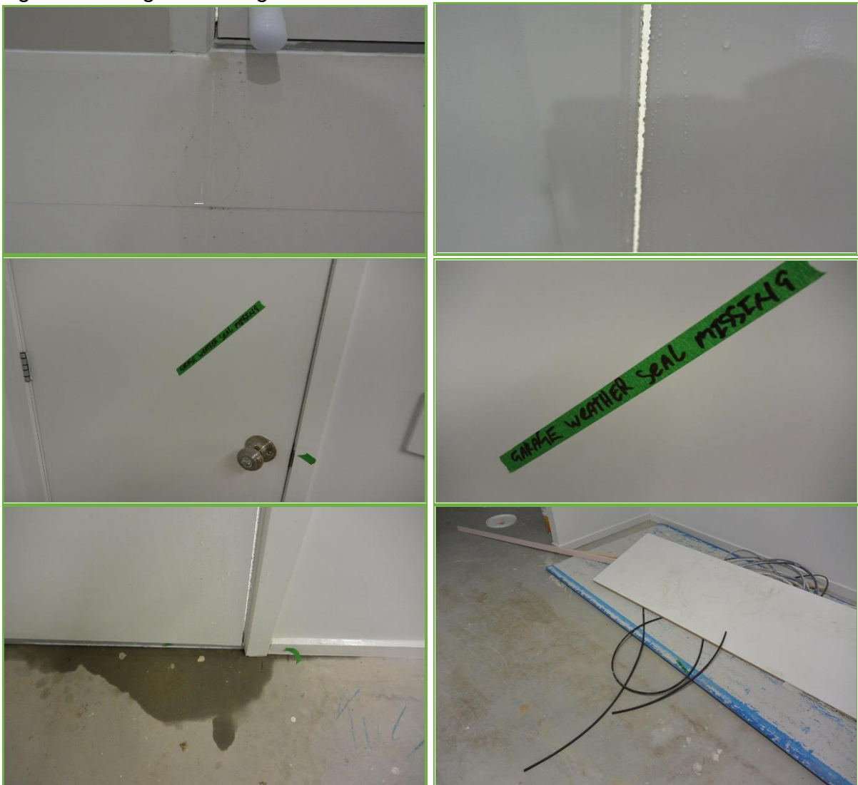
Allowing water to ingress during rain
