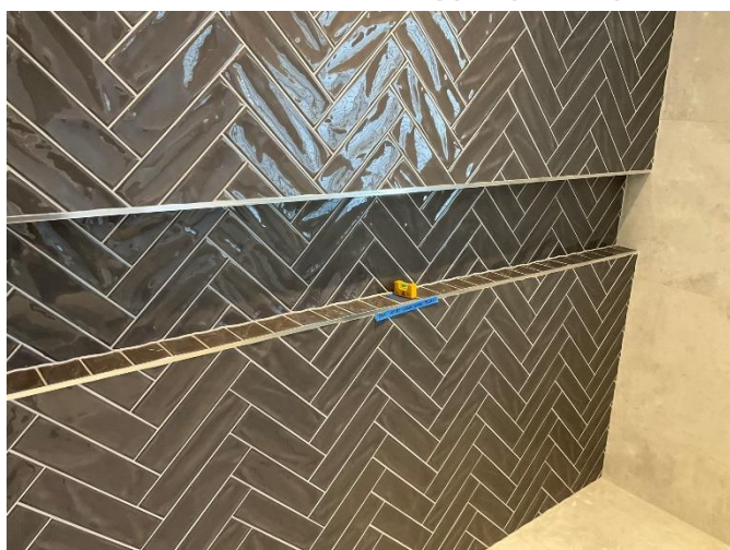
FIGURE 3.4 TYPICAL DETAIL FOR RECESSED SOAP HOLDERS
