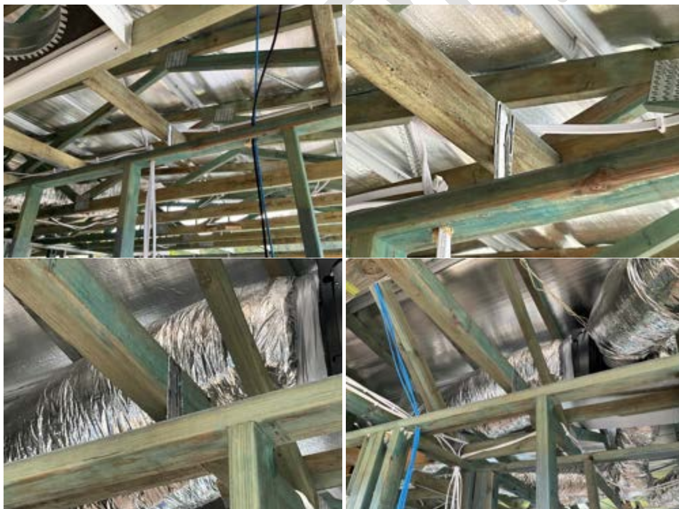
FIGURE 2.3 FIXING OF TRUSSES TO FREESTANDING NON-LOADBEARING WALL THAT IS NOT A BRACING WALL
