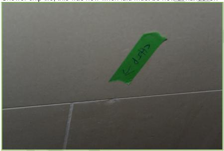
5. Voids in grout in main bathroom, this will need re-work before handover.
