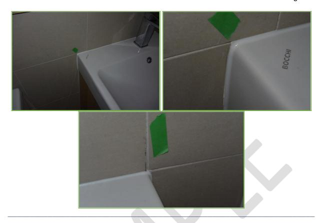
1. Bathroom slider door margins are uneven this will need re-work before handover.
