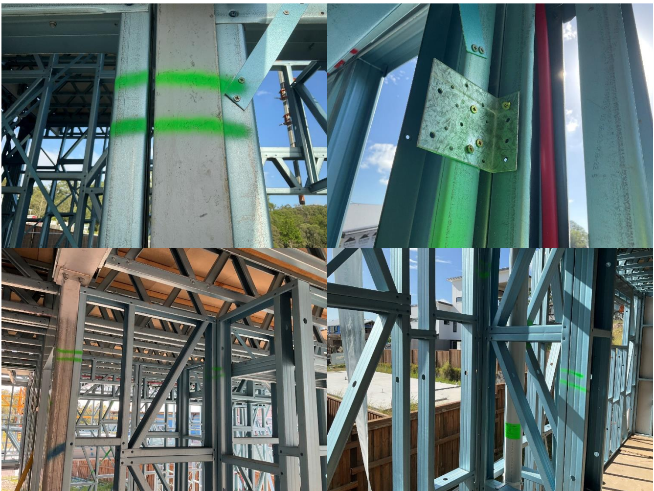
Fig. 3.5 Corners and junctions showing examples of stud positions and fixings
